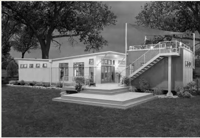
▲ Figure 3-7 The roof of the one-bedroom unit (left) accommodates rainwater harvesting; the flex room (right) is shown with a roof deck. Image courtesy of Clayton Homes.
