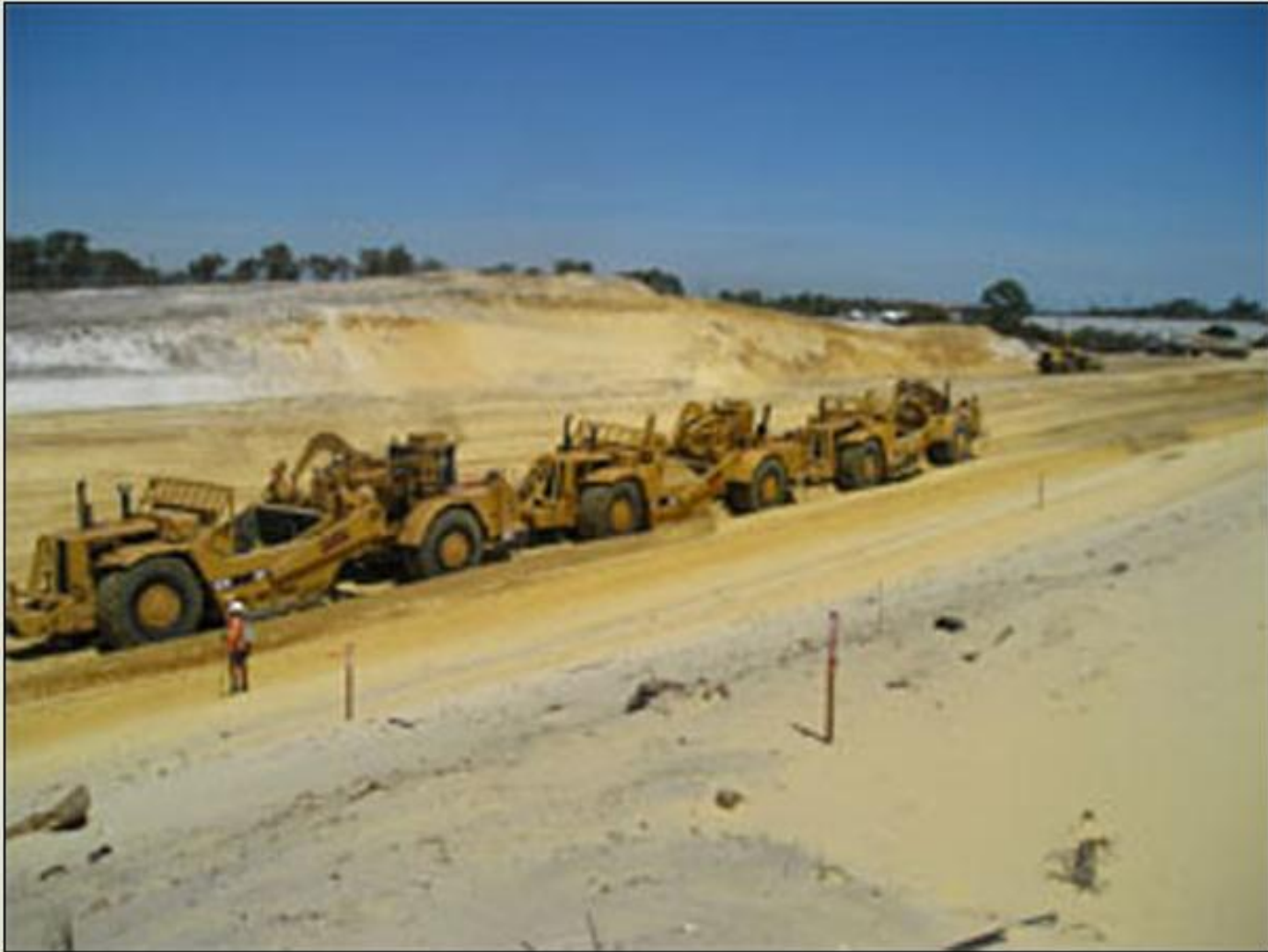
Push-pull scrapers March 2005
